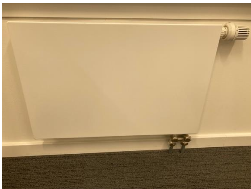
35- radiators with conventional thermostats
